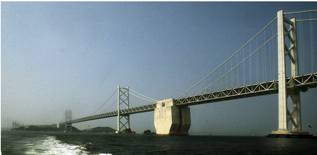
Fig. 2 - Kita Bisan-seto/ Minami Bisan-seto 1987. Double suspension spans 990 m and 1100 m.
