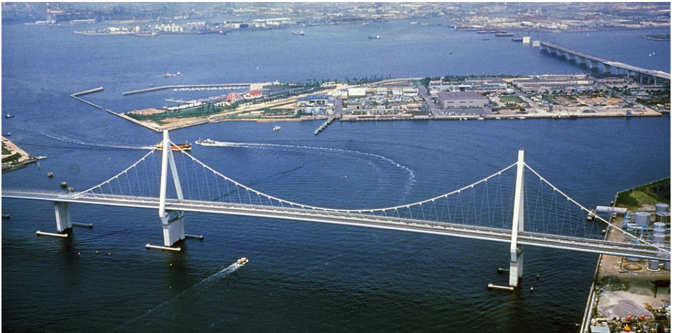
Fig. 1 - Konohana Bridge - Osaka, Japan - 1990. Monocabre suspension span - self anchored cables - box deck.
