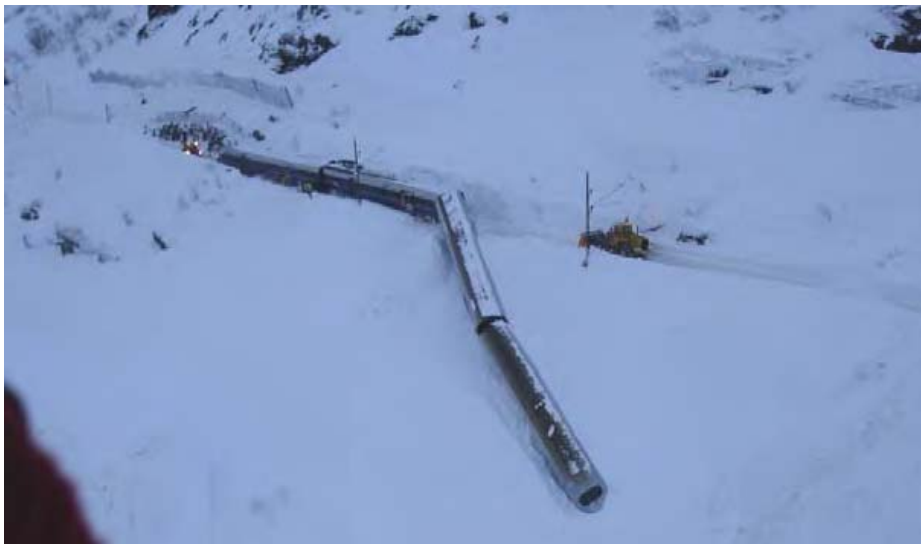
Figure 38. The train derailed with two cars between two over-head wire poles without striking them. The pantograph, located on the third car of the four car set, was in contact with the over-head wire also after the derailment. The second train unit has been moved backwards before the photo was taken. 27
