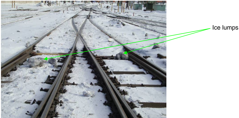
Figure 62. Ice lumps fallen off in a yard from low speed passing trains close to switches.
