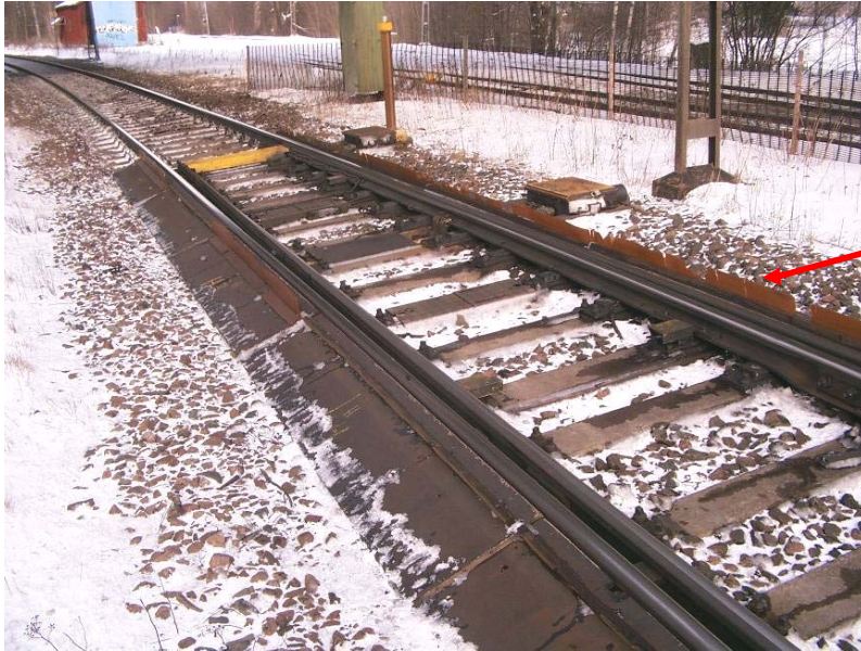
Figure 53. Skutskär. A main line switch with a rubber spoiler as well as a cover outside the rails. Notice that there are double motors for altering the switch. 44
