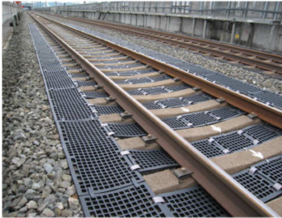
Figure 66. Ballast screen at East Japan Railway Company with a quick-release ballast screen for effective maintenance 55 .
