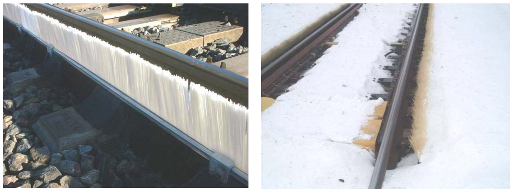
Figure 54. Detail of a brush spoiler is seen to the left. To the right the mounting outside the main rails in a switch is shown. 45
