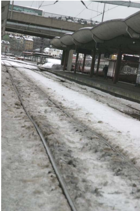
Figure 61. A platform track with a lot of ice that has fallen of stopping trains at a main station.
