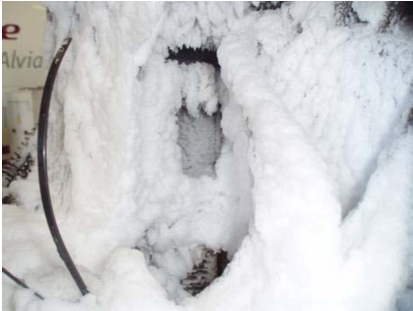
Figure 11. A Talgo running gear subject to snow and ice build up during a winter test. 10
