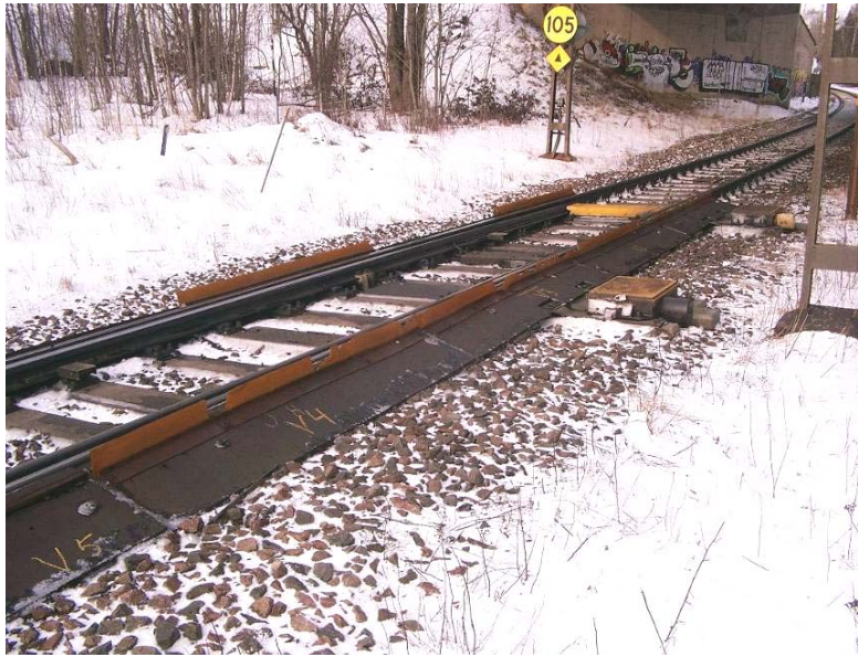
Figure 55. A switch with rubber spoiler and covers outside the main rails. The contacts for positioning control of the tongue can be seen next to the far tongue. 46
