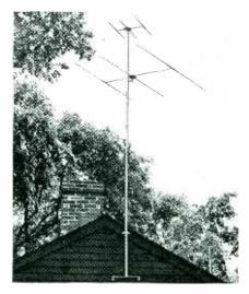
on a single mast and designed for reception of all channels operating in a particular area. Elements are constructed of half-inch aluminum tubing. More arrays can be added to the installation as additional stations go on the air.
