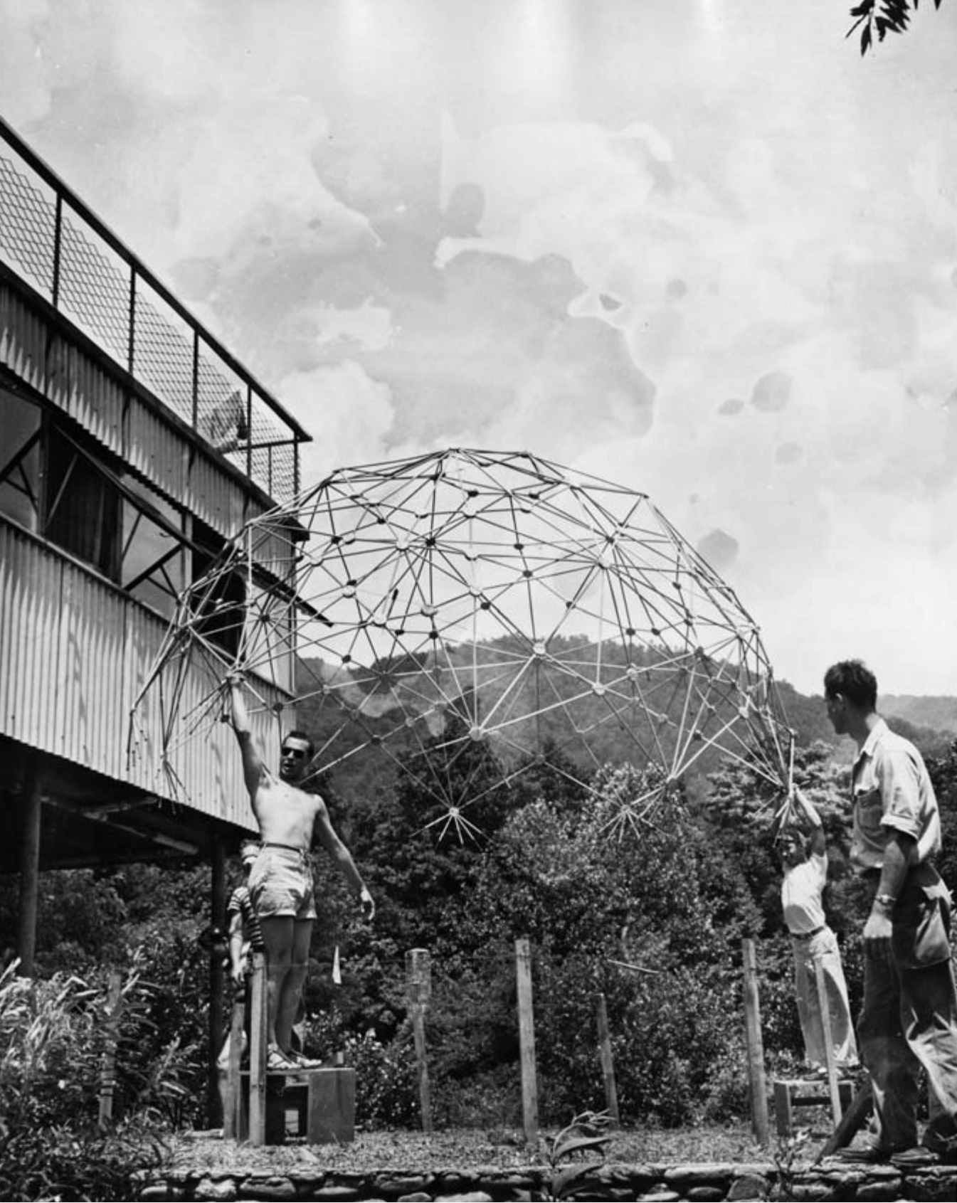
Figures 3.9 (previous page) and 3.10 (above) Masato Nakagawa, Buckminster Fuller's dome of thirty-one great circle necklace structure of tubular beads and continuous internal cable with double heat-sealed, pneumatic, transparent skin. Designed
