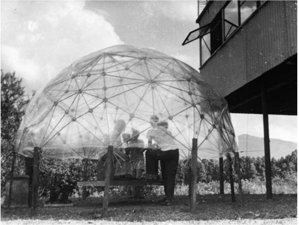
Figure 3.12 Masato Nakagawa, Buckminster Fuller's Dome, Demonstration of Plastic Skin . Black Mountain College, summer 1949. Courtesy of the State Archives of North Carolina.
