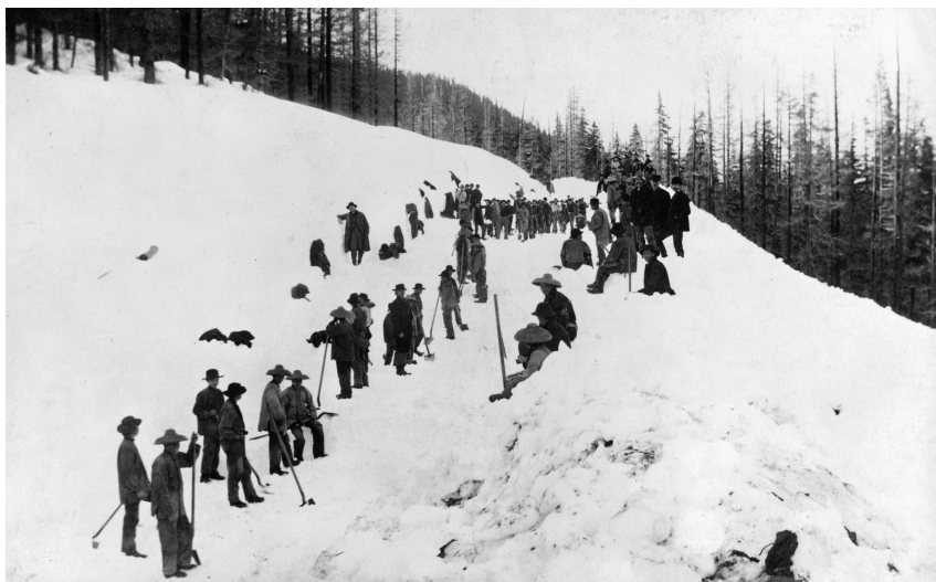
FIGURE 1.4 Chinese workers clearing snow from railroad tracks, 1886. Heavy snowfall sometimes buried tracks so deep that rotary snowplows could not operate. Then it was necessary to employ shovel gangs to clear tracks. University of Washington Libraries, Special Collections, UW552.
