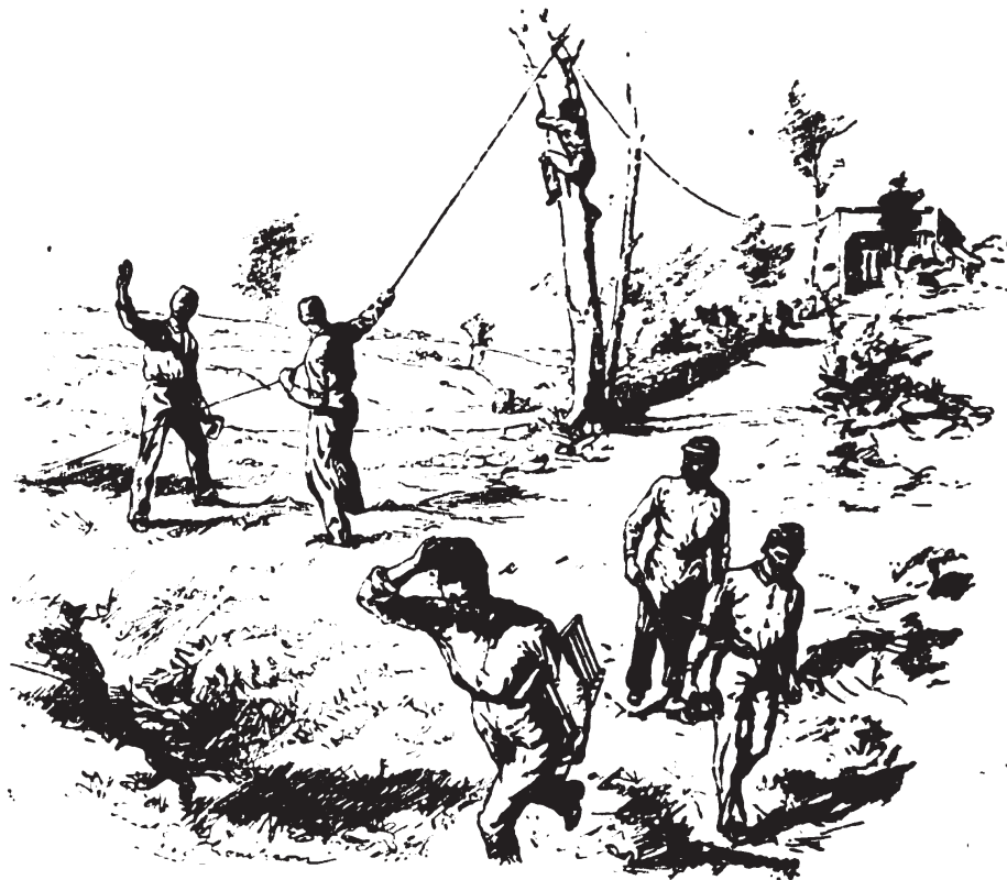
Running the Wires of a Field-telegraph.
