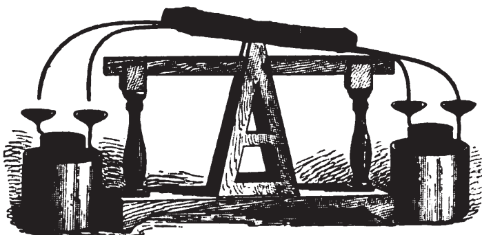
Professor Joseph Henry's Electro-magnetic Motor. (From a photograph of the original.)
