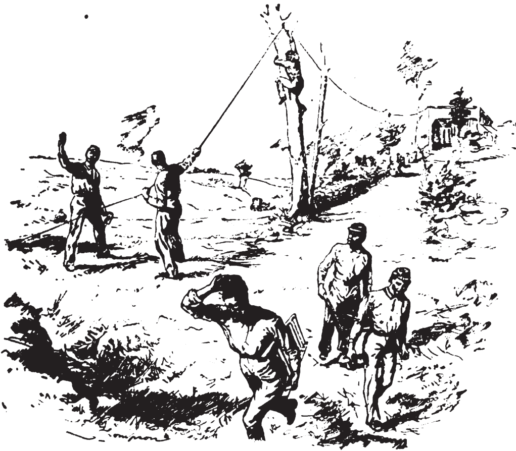
Running the Wires of a Field Telegraph.
