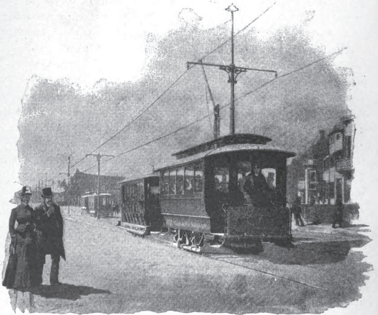
Fig. 4.—Overhead Wires for Double-track Road, suspended on a Single Line of Ornamental Poles.— Thomson-Houston Railway, Washington, D.C.
