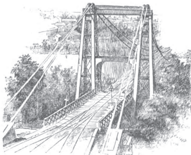
The New Iron Towers of the Same
