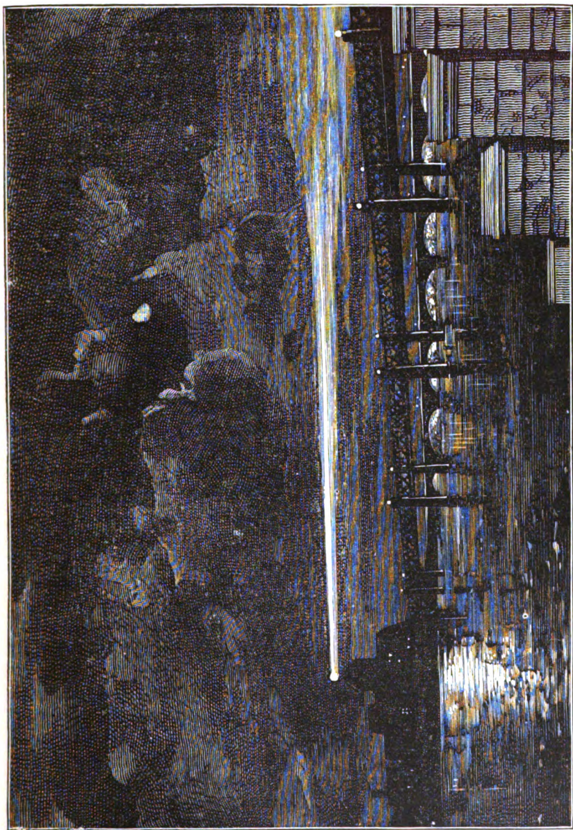
FIG. 147.—Experiments in the projection of the electric light at London, on the Thames, with a Brush lamp of six hundred curcels.
