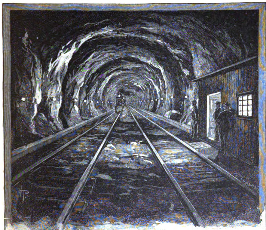
Fig. 22.—The Hoosac Tunnel Lighted by Glow Lamps.
