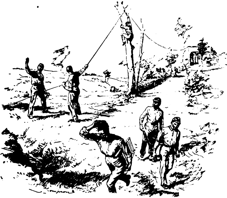
Running the Wires of a Field Telegraph.
