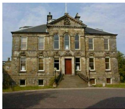
1. Cumbernauld House, the Elphinstone-Fleeming family residence, designed by William Adam and erected in 1731, near the site of the large castle built by the Fleemings or Flemings at the end of the 14 th century ..
